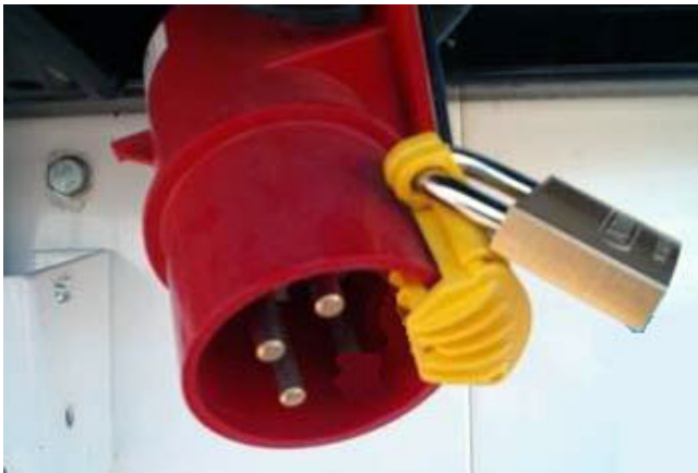
Figure 2 - Lockout/Tagout Device
